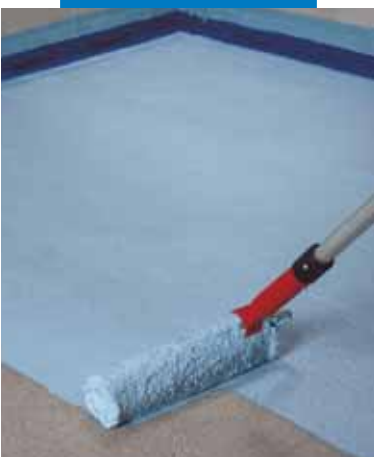
Application of the first coat of Mapelastic® AquaDefense on a screed
