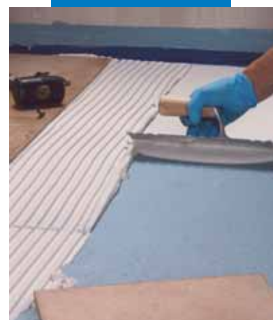
Bonding tiles on Mapelastic® AquaDefense
