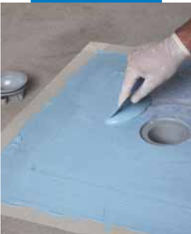
Impregnating Drain Vertical fabric with Mapelastic® AquaDefense
